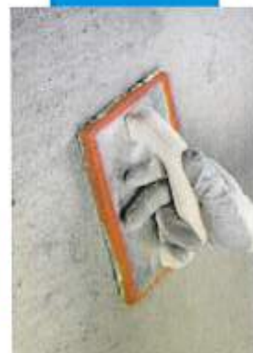
Tamping Planitop Smooth & Repair
