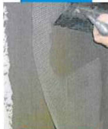
Smoothing insulating panels reinforced with a Fibreglass Mesh: dropping into the coat of Mapetherm AR1
