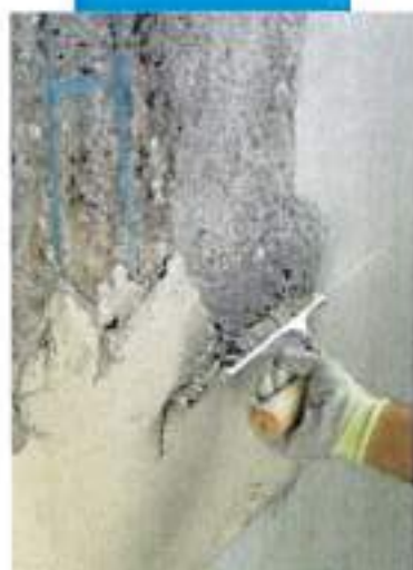
Application of Planitop Smooth & Repair with a spatula
