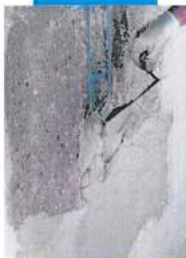
Application of Planitop Smooth & Repair by trowel
