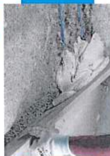
Smoothing of Planitop Smooth & Repair with a straight edge
