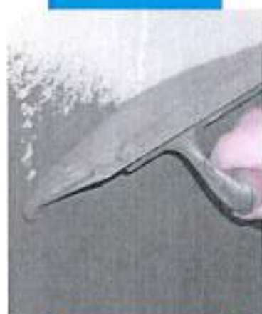
Smoothing insulating panels: spreading the Mapetherm AR1
