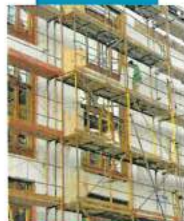
Bonding the insulating blocks to the facade with Mapetherm AR1
