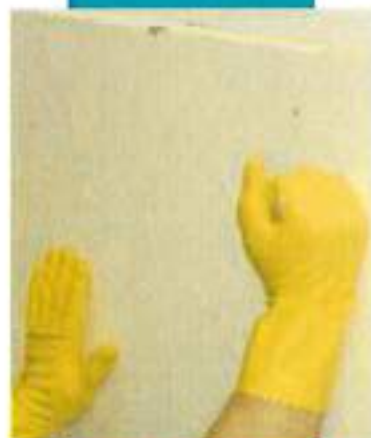
Applying pressure on the panels once they have been installed. This is to ensure a good bonding to the surface
