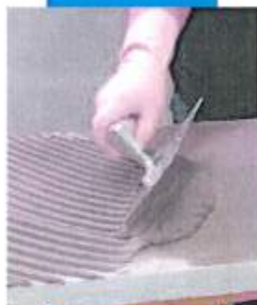
Applying Mapetherm AR1 on the back of the panel with a notched trowel
