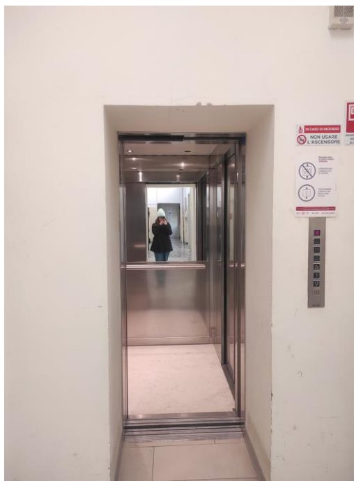
Photo 2: Elevator entrance, the side walls measure 80 cm
